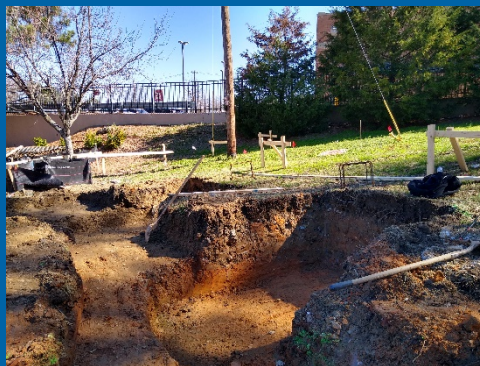
Begin Excavation for Canopy and Retaining Wall Footings
