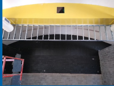
Install Drywall Framing at STEM Lab
