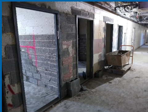
Installation of Door Frames in Masonry Walls
